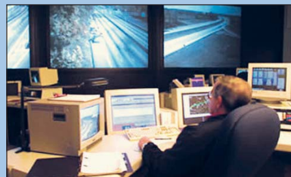
The Northern Virginia Smart Traffic Center, run by the Virginia Department of Transportation, monitors traffic flow on over 100 miles of roads.
