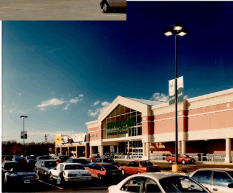
Penn Mar Shopping Center "After" Renovation with new Super*Fresh Anchor
