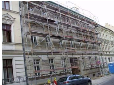
Conservation-Protected House, Berlin-Köpenick – during modernization
