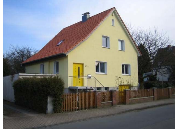
One-/Two-Family Home, Hanover – after modernization
