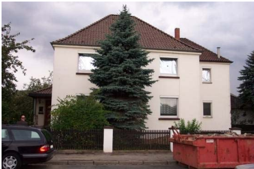
Single-Family Home, Bruchstrasse, Ronnenberg – before modernization (left)
