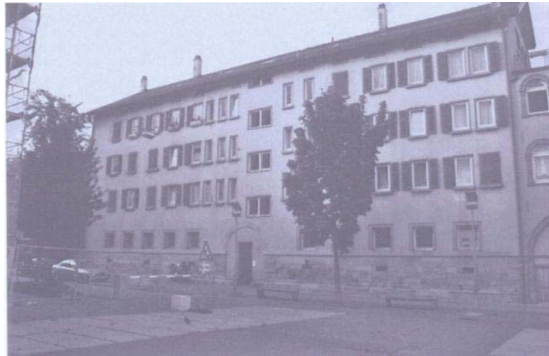
Guesthouse for Young People, Kanalstrasse, Esslingen am Neckar – before modernization
