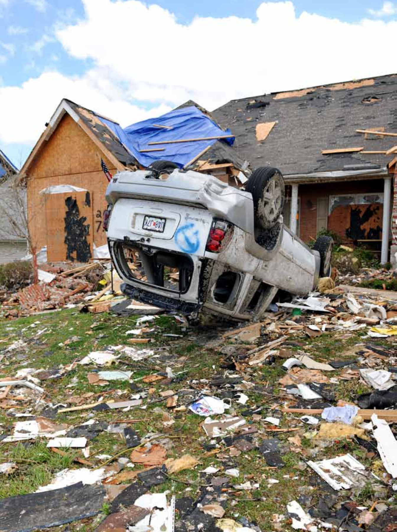
Saint Louis, Missouri - Destroyed homes after tornadoes, Saint Louis area on Friday April 22, 2011. Photo: © R. Gino Santa Maria | Dreamstime.com
