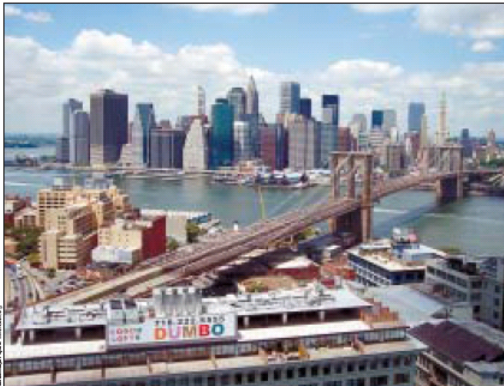
This is the $2.4-million view from the 1,300-square-foot penthouse of the Beacon Tower at 85 Adams St. In DUMBO. The 297-foot, 23-story tower is the largest (so far) to go up in the rapidly developing neighborhood.
