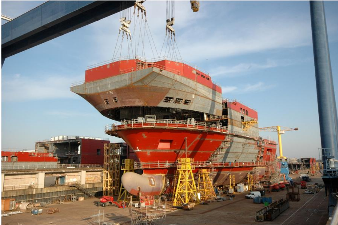
Figure 8. Example of the modular construction of the Mistral BPCs. This is the 690 ton forward module being assembled for the third French BPC, the Dixmude . (From Bernard Biger, STX France, 2009) 76
